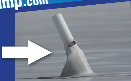
above: Vent damage from typical snow loads
