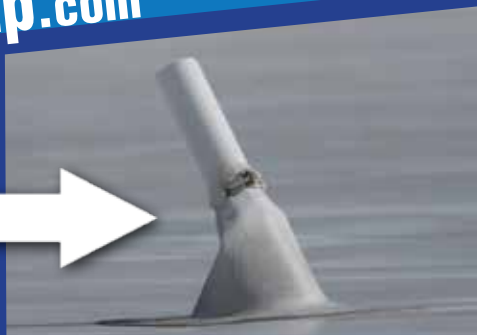
above: Vent damage from typical snow loads
