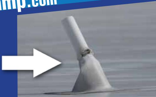
**above:** Vent damage from typical snow loads
