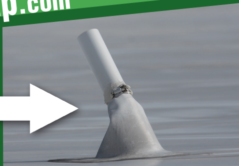
above: Vent damage from typical snow loads
