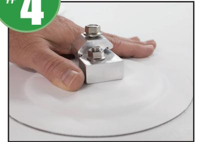
Lift the elastomeric flange and install eight additional fasteners through the MCP steel plate, hitting the top flutes in the deck. *Do not fold or crease the membrane during fastener installation.*
